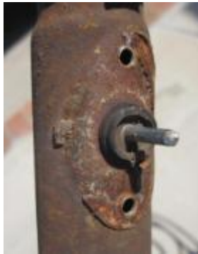
Pin and grommet in place
